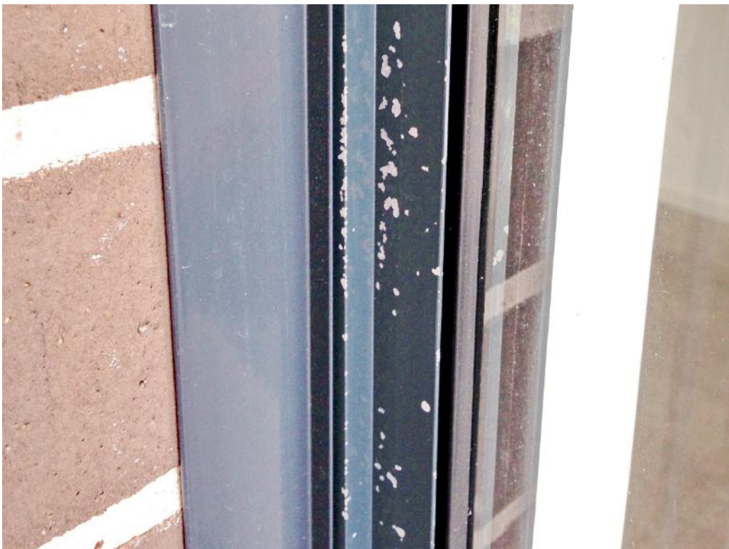
Appendix B: Examples of powder coating that has failed in the field after less than 6 months. Coated by another coater who does not have proper, nor Qualicoat Standard Pre-treatment for Aluminium.
